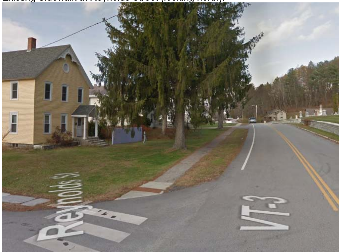
Existing Sidewalk at Reynolds Street (looking north):
