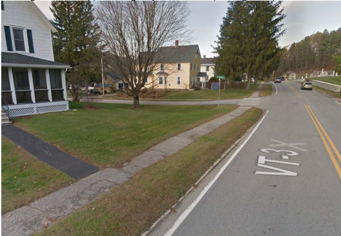
Existing Sidewalk Approaching Reynolds Street (looking north):
